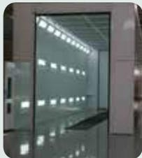
Overspray and fumes are extracted through ducts in the floor, into a filtration system that captures all the paint particles and only then is the air expelled into the atmosphere.
